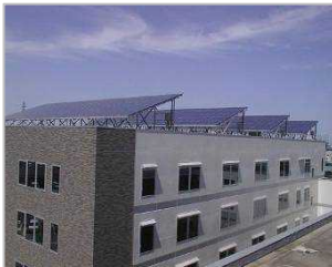
Solar Panels at New Headquarters
