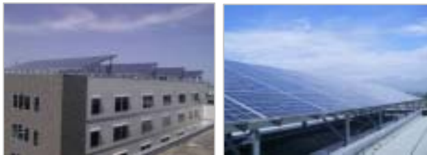
Solar Panels at New Headquarters Solar Panels at Tateyama Plant
