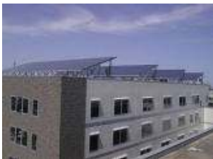
Solar Panels at New Headquarters
